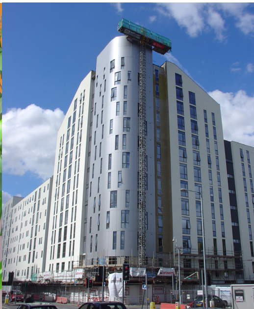
Left to right: Dragana Opačić and her projects Plymouth Grove mixed use scheme, Manchester and grade 2* listed, South Manchester Synagogue.
