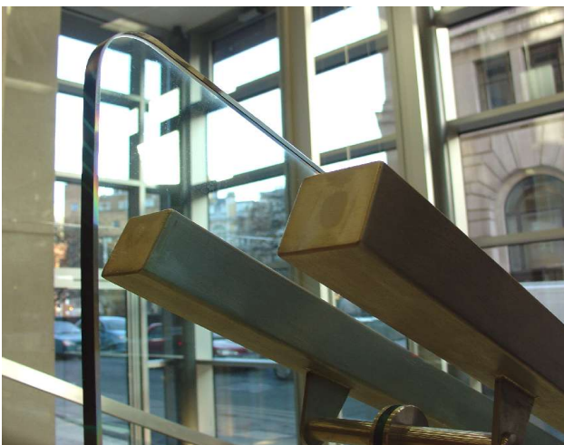
Above: The new glass entrance with the glass and brushed steel balustrade in the foreground
