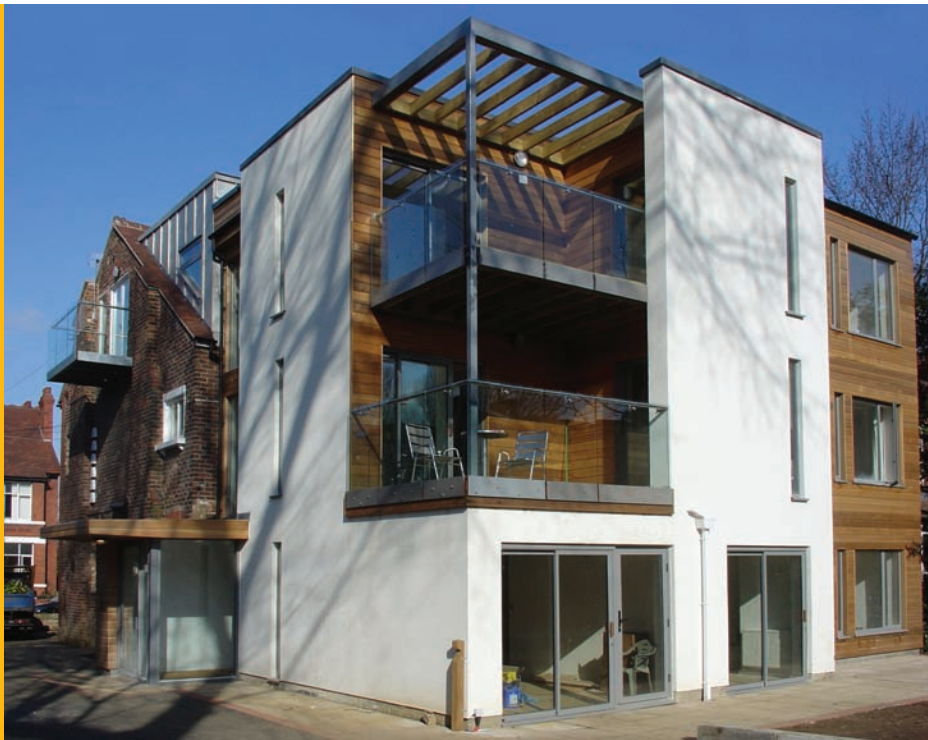
Above: Moorfield Street, West Didsbury, rear/side elevation.
