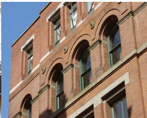
Left: Amazon House, Brazil Street, interior and exterior.
